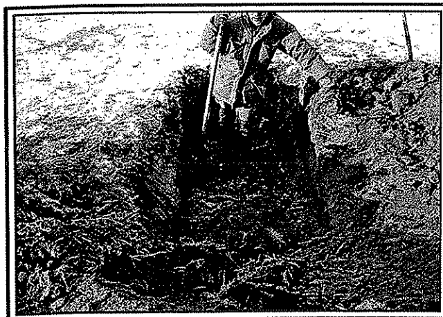
Photograph 5. View to the south showing one of the wider backhoe tests excavated.
