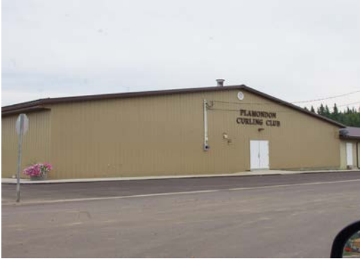
Curling club 101 Avenue and 98 Street
