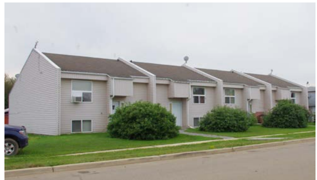
Fourplex south side 100 Street between 98 & 99 Streets
