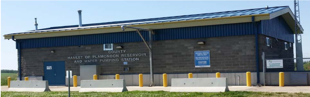
Pumphouse, reservoir and truck fill
