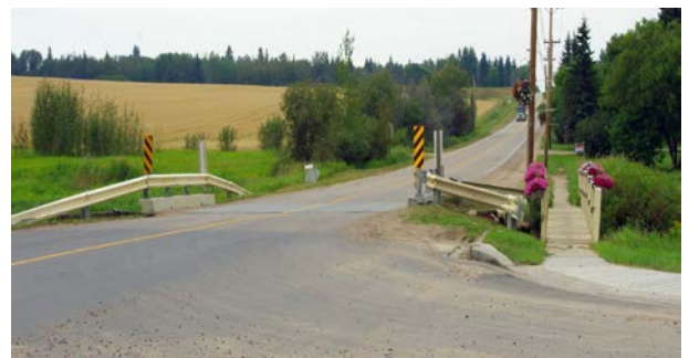
100 Street bridge crossing Plamondon Creek looking north
