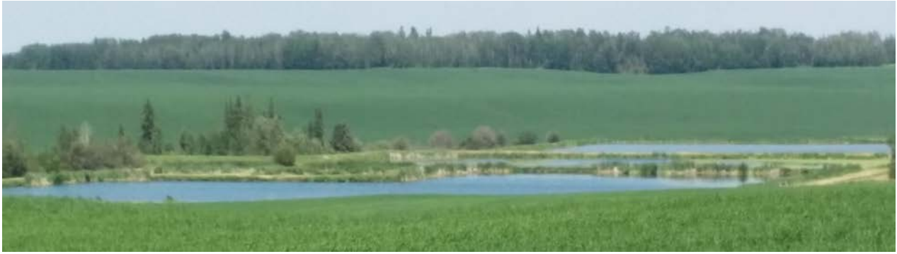
Aerobic Cells and Anaerobic Cells of the lagoon system, northeast of the urban area
